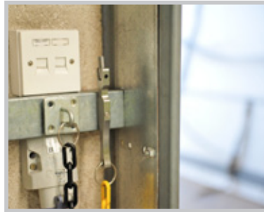
2. SafeLoader is operated with specially designed key, housed on the loading bay.
